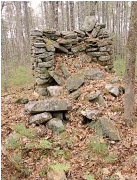
Collapsed firebox
