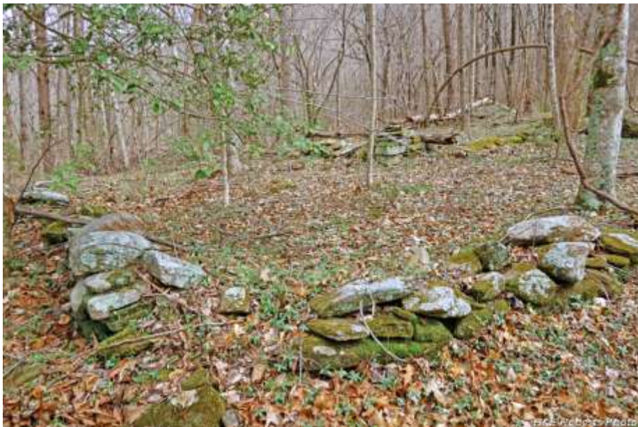
Stone enclosure surrounding a foundation & collapsed chimney
