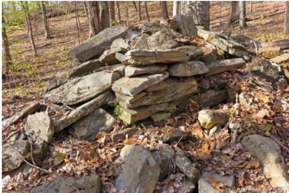
Collapsed chimney pile
